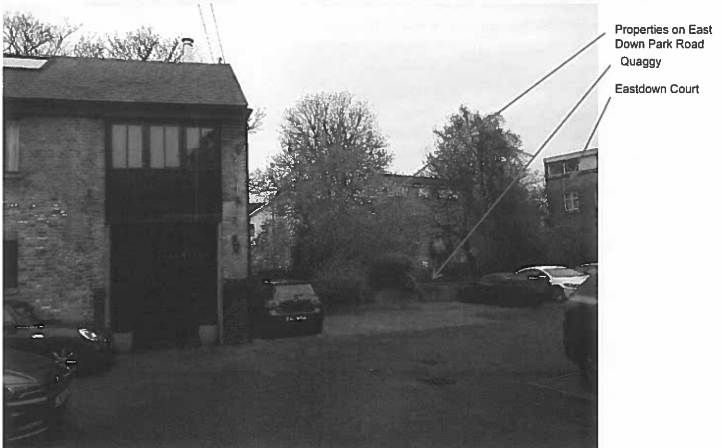
Photo 7: View towards the Quaggy river bank, No 17 Waterside Court and houses on the Eastdown Park road from Waterside Court carpark (photo taken on 23.03.2019)
